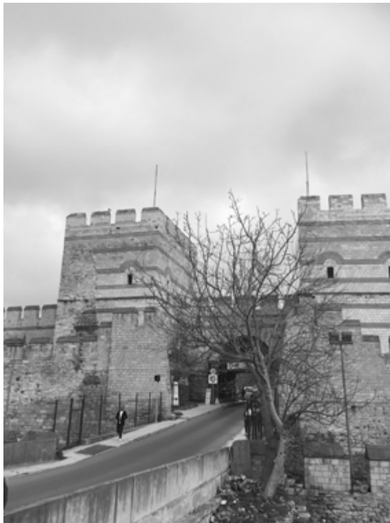
Fig. 3. The current state of the Belgrade Gate. Photo by Olof Heilo 2019.
