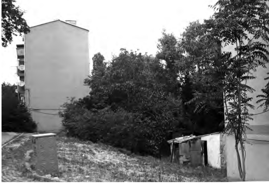
Fig. 4. An informal extension in the open space between the blocks. Photo by the author.
