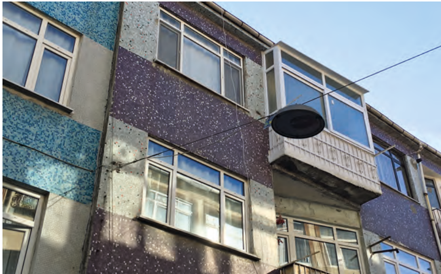
Fig. 7. Glass mosaic façades at Melek Hoca Caddesi. Photo by the author.
