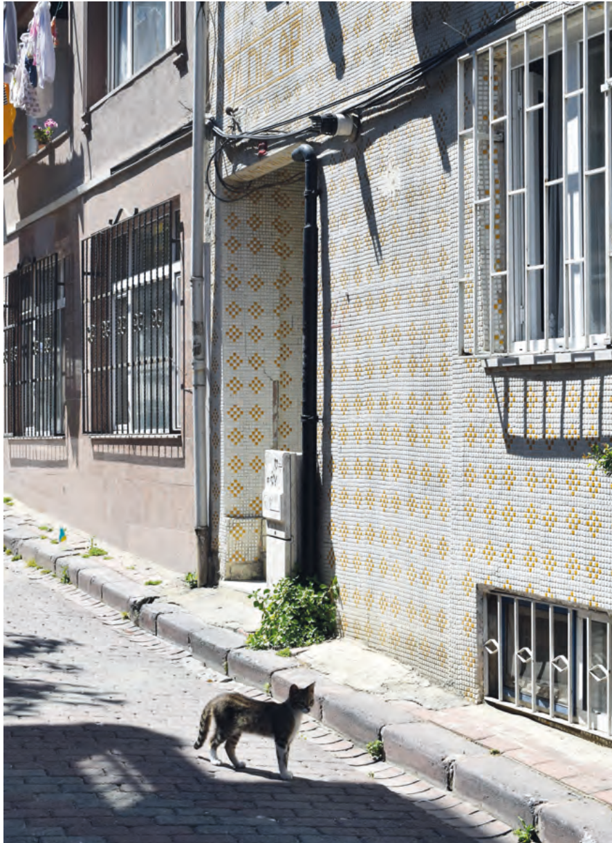
Fig. 10. Street in Ayvansaray, Balat. The façade is clad with 10x10 mm machine-made mosaic pieces. Photo by the author.
