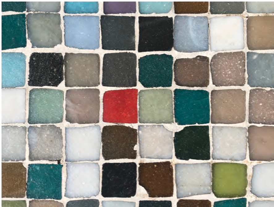
Fig. 2. Detail of hand-cut glass mosaics from the 1960s in the size of 20x20 mm. Photo by the author.
