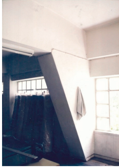
Figure 8a and 8b. Block 7495 in 1998: opening in the shop's ceiling in 7495/2 (a), a gusset with an enormous size on the first floor of 7495/1 (b).
