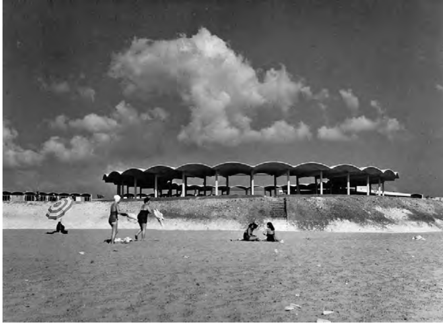
Fig. 4. Florya Camp and Beach Facilities designed in 1956–1959 by Sedad Hakkı Eldem with Orhan Çakmakcioğlu. Rahmi M. Koç Archive © Pera Museum, (catalogue Istanbul's Seaside Leisure 2018).
